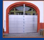
With beams weighting less than 8 kg per meter, single handed installation is possible within safety guidelines for lifting.
