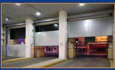
Because of the demanding requirements in terms of reliability, drop down barriers are normally designed to be fully automatic. Manual operation, e.g using a dead man's control, is also possible. The ideal solution for danger areas that must be protected of sudden floods through heavy rain
